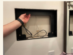
Original Wall Cavity
